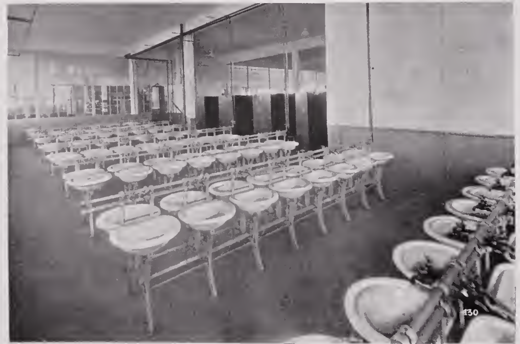
"CLEANLINESS NEXT TO GODLINESS" No Unnecessary Waiting to "Wash Up"
